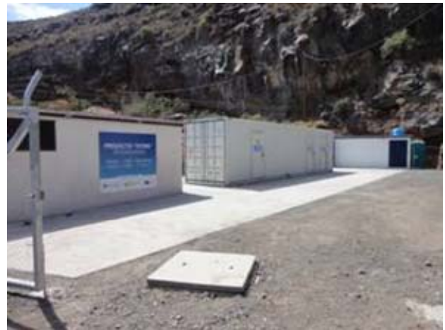
Figure 5: Installation of La Gomera flywheel
