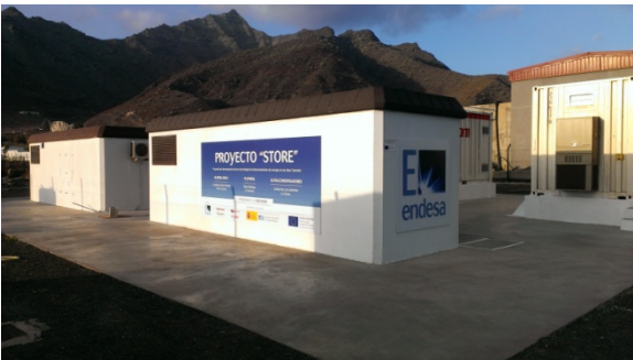
Figure 8: Installation of Gran Canaria battery.
