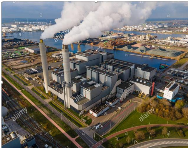
Figure 17 Waste recovery plant
