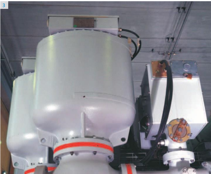
1 Circuit-breaker | 2 Disconnectors/earthing switches | 3 Voltage transformer and fast-acting earthing switch | 4 Connecting elements | 5 Control & protection
