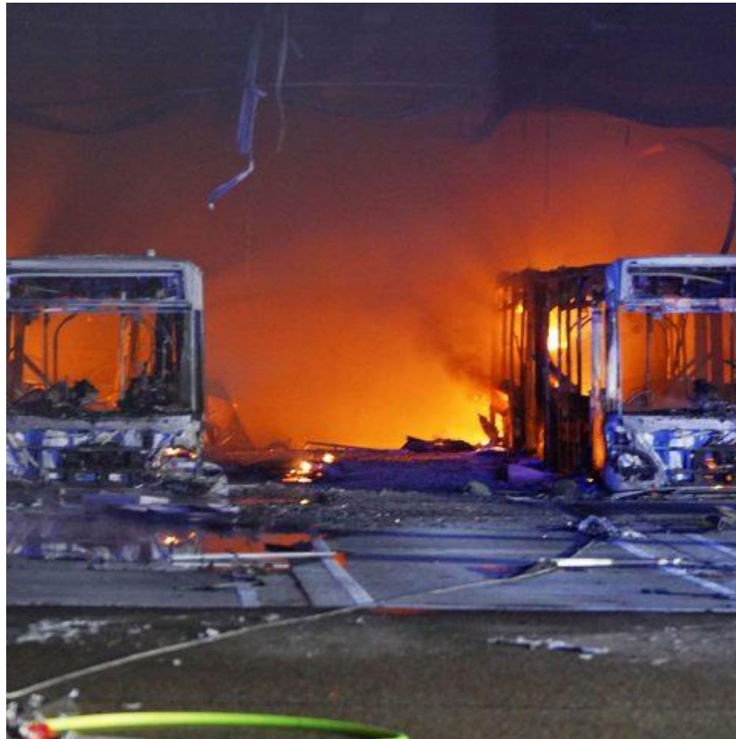
Figure 15: Fire at the Gaisburg bus depot in Stuttgart, with multiple buses affected [SUST21].
