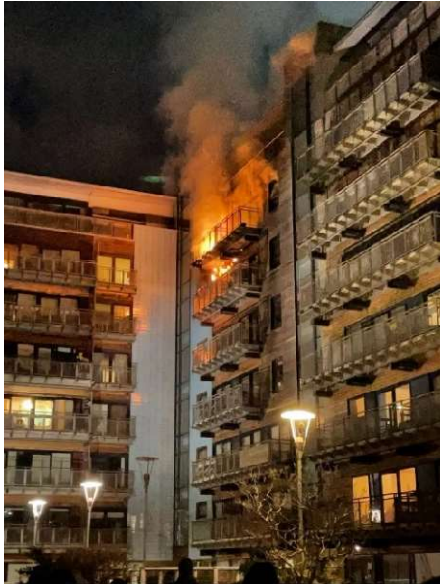
Figure 19. Vertical spread in residential fires a) [54] b) [55].
