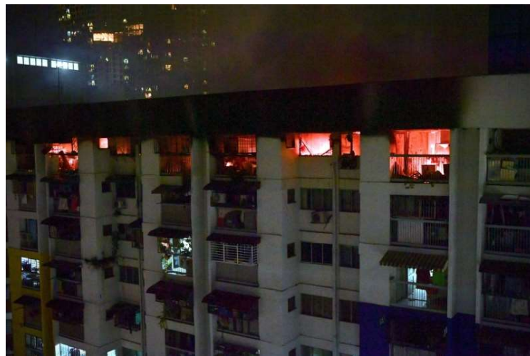
Figure 18. Horizontal spread in residential fire [60].
