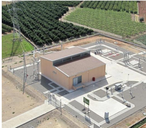
Figure 129: Remote office (Source: Iberdrola)
