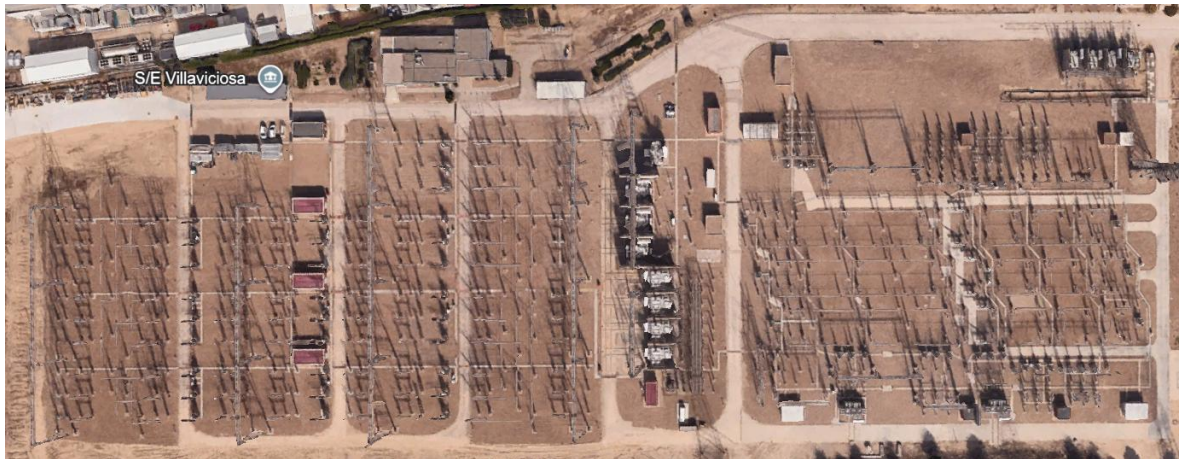
Figure 2. Villaviciosa de Odón substation [GOOG26]
