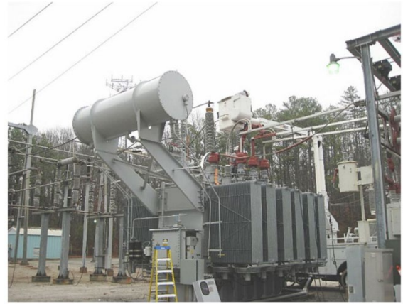
Fig. 1. TDSF monitoring in a 230 kV/20 kV, 60 MVA distribution substation transformer.
