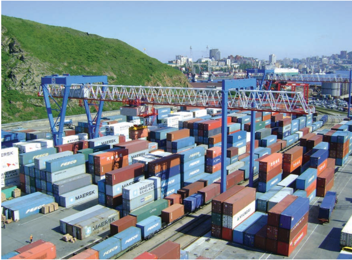
Fig. 3.9: Rail Mounted Gantry Crane
