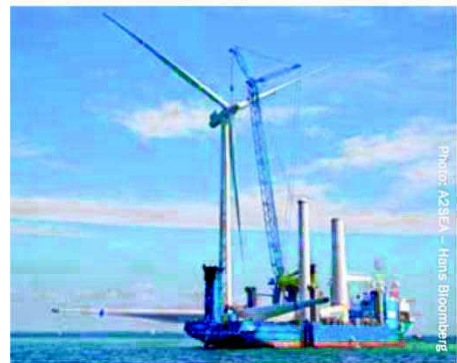
Leg-stabilised crane vessel
