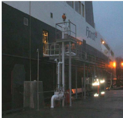
Figure 3 - PTS bunkering Source: GASNOR
