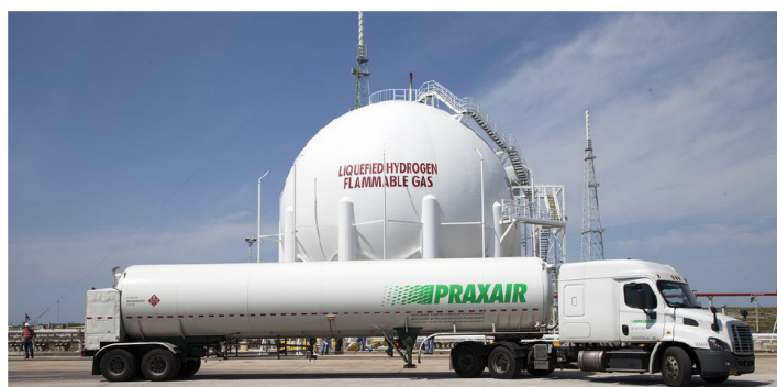
Figure 2.13. Liquefied hydrogen transport and storage.
