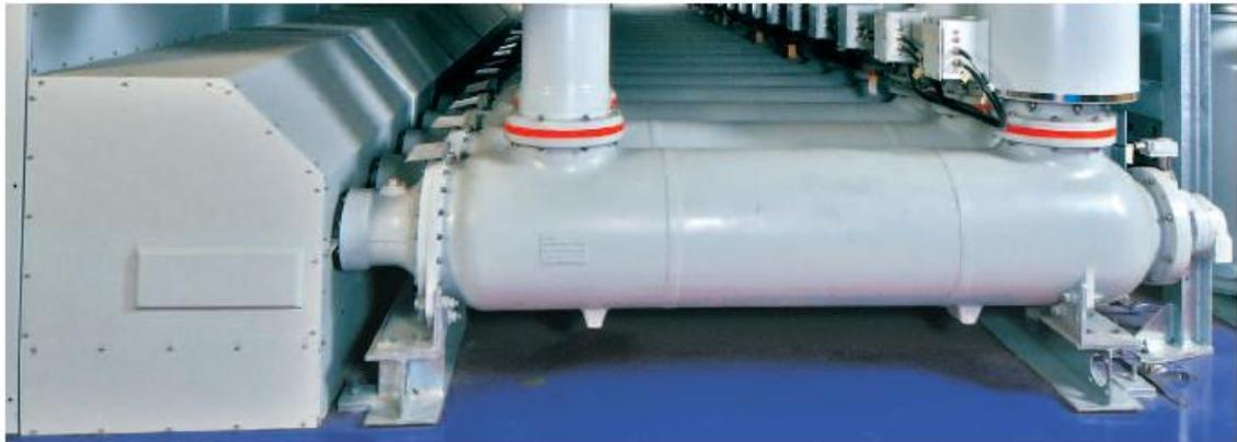
Circuit-breaker with operating mechanism
