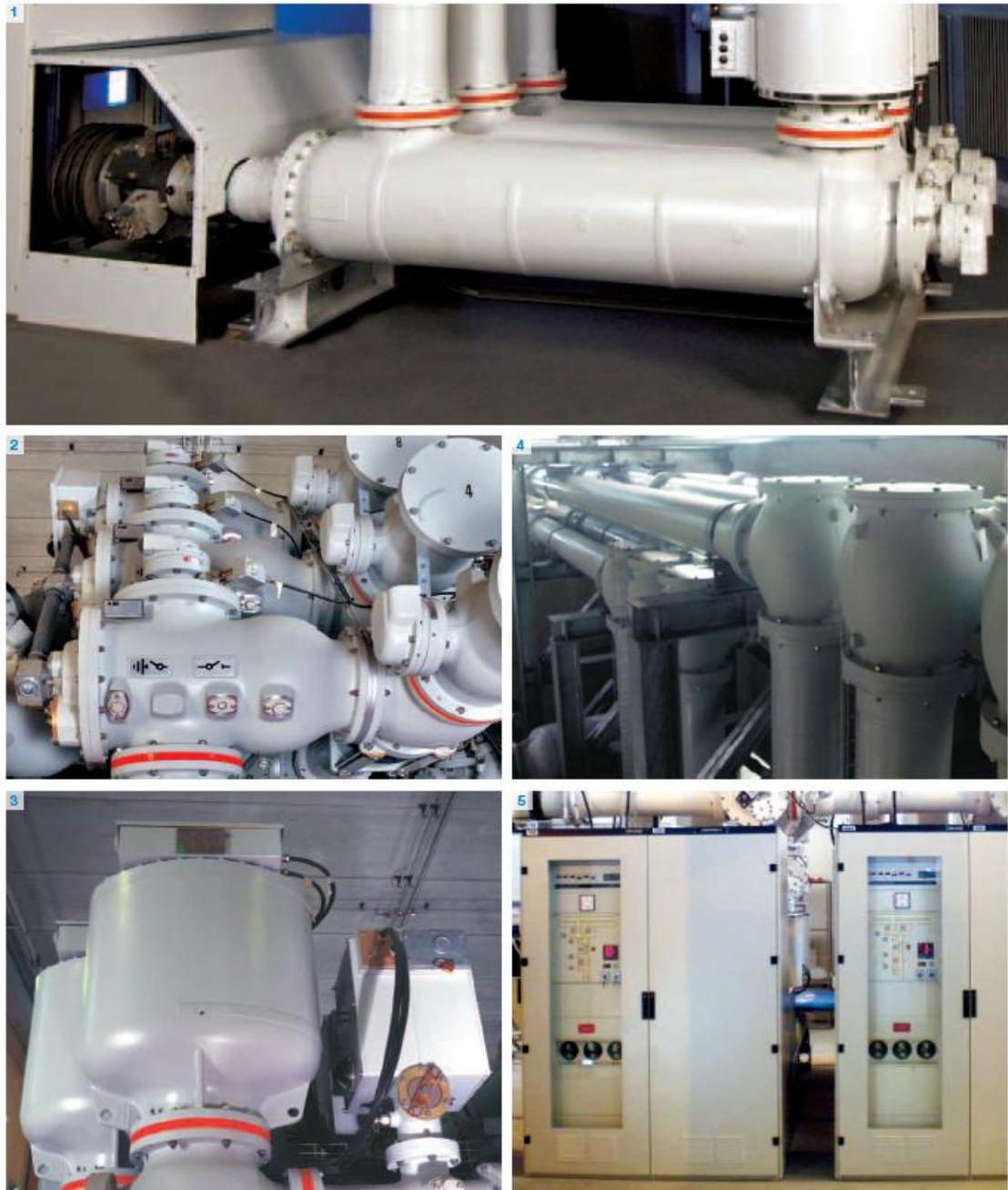
1 Circuit-breaker | 2 Disconnectors/earthing switches | 3 Voltage transformer and fast-acting earthing switch | 4 Connecting elements |
