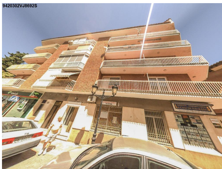
Illustration 1. Building facade. Source: National Cadastre
