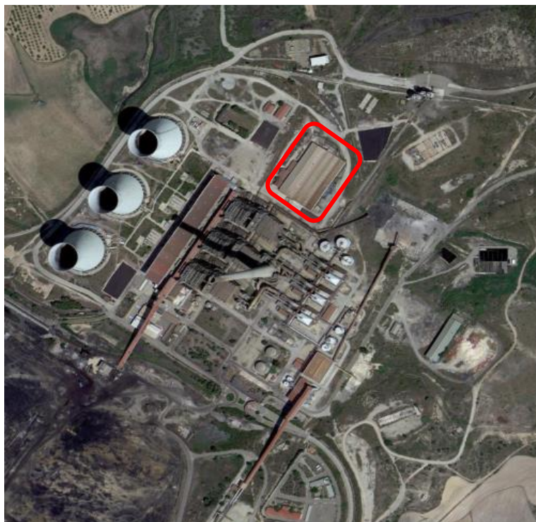
Figure 3 Old thermal power plant in Andorra.
