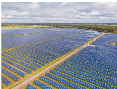
Figure 2. Solar PV plant in Spain
