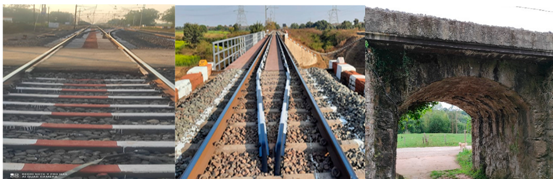
Figure 3. Check rail (left). Guard rail (centre). Supporting track walls for ballast contention (right).
