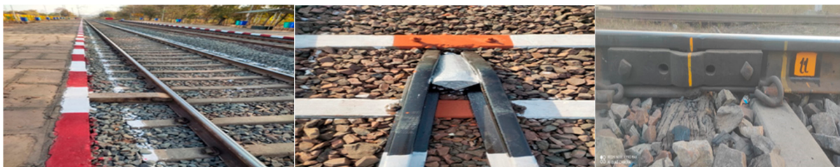
Figure 9. Blocks made from wooden sleepers used to maintain the rail's distance from the platform (left), to keep the separation between guard rails at the end of adjacent sides to grip well and erode less (centre), and to support and absorb wheel impact under fishplate joints at welded sections.
