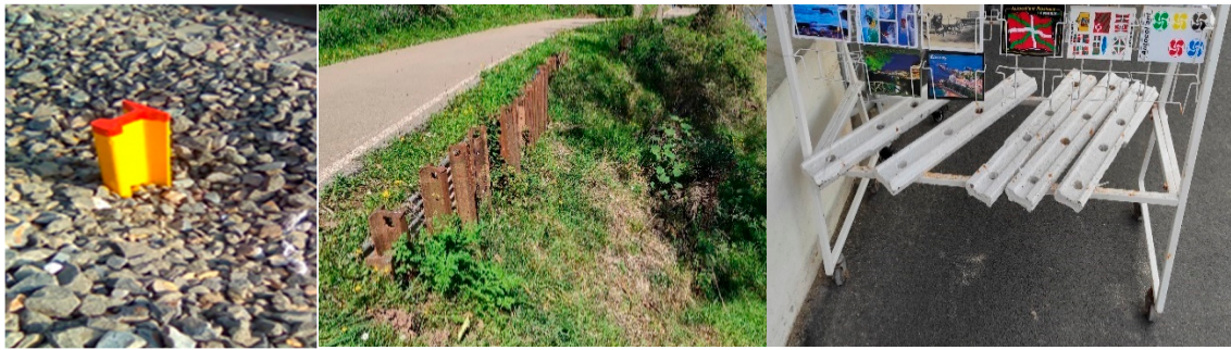
Figure 4. Rail pegs (left). Slope stabilisation with rails (centre). Fishplates for supports (right).
