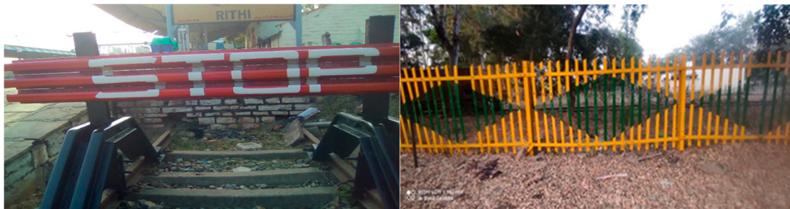
Figure 2. Dead end (left). Rail fencing (right).
