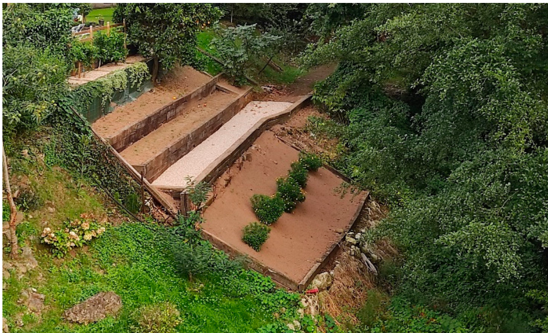
Figure 10. Slope stabilisation with second-hand wooden sleepers.
