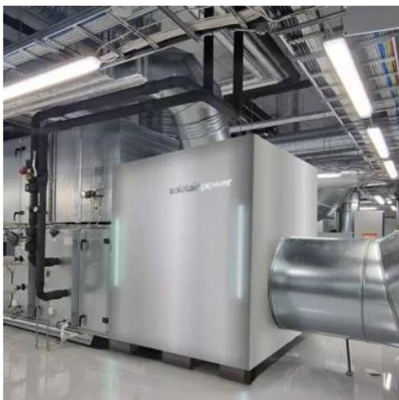
Figura 18: Módulo DAC-HVAC de Soletair Power [37]
