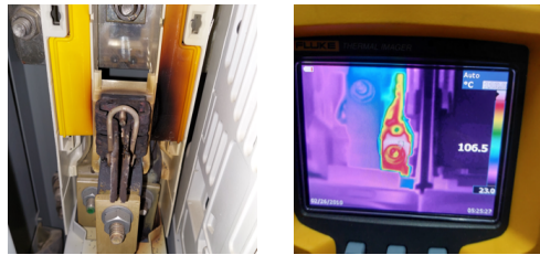
(a) Damage caused by a hot spot event detected in a routine maintenance (b) Thermal imaging of the hot spot event
