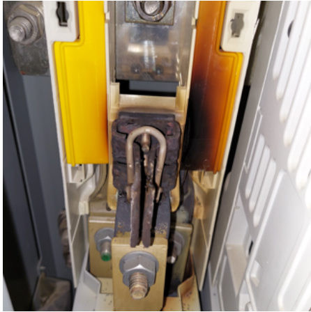
(a) Damage caused by a hot spot event detected in a routine maintenance
