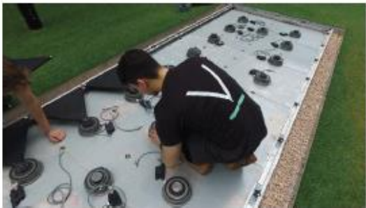
The GRP base is secured in place with masonry anchor bolts.
