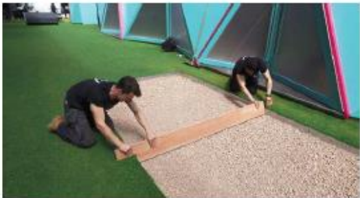
Local construction team excavate and prepare site. The Pavegen team then lays screed base and levels to a 92mm depth.
