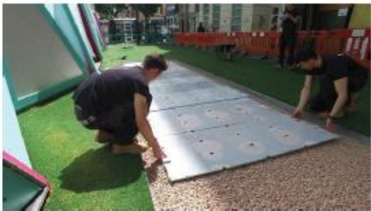
Glass reinforced plastic base is laid and interlocked for a durable surface.
