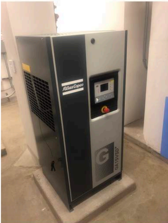
Figure 4: Secondary air compressor
