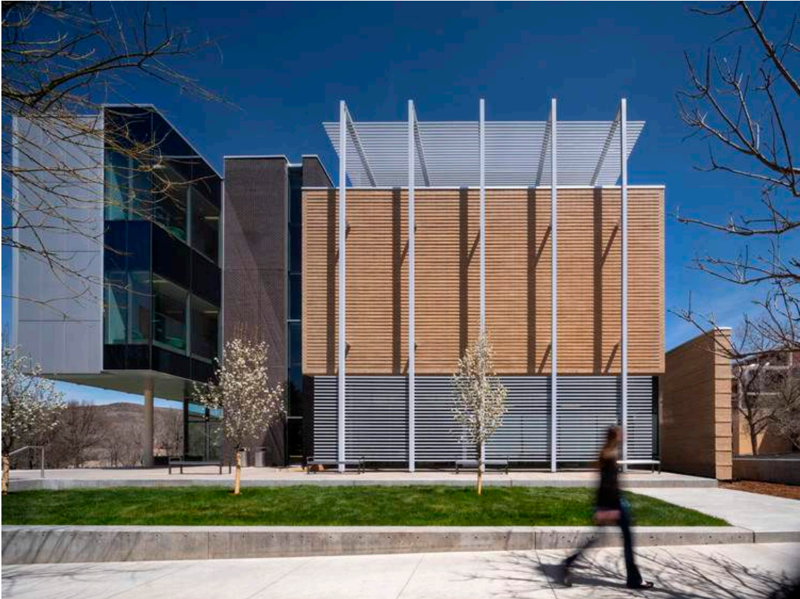
Photo 5: CoorsTek center from Illinois Street – East elevation
