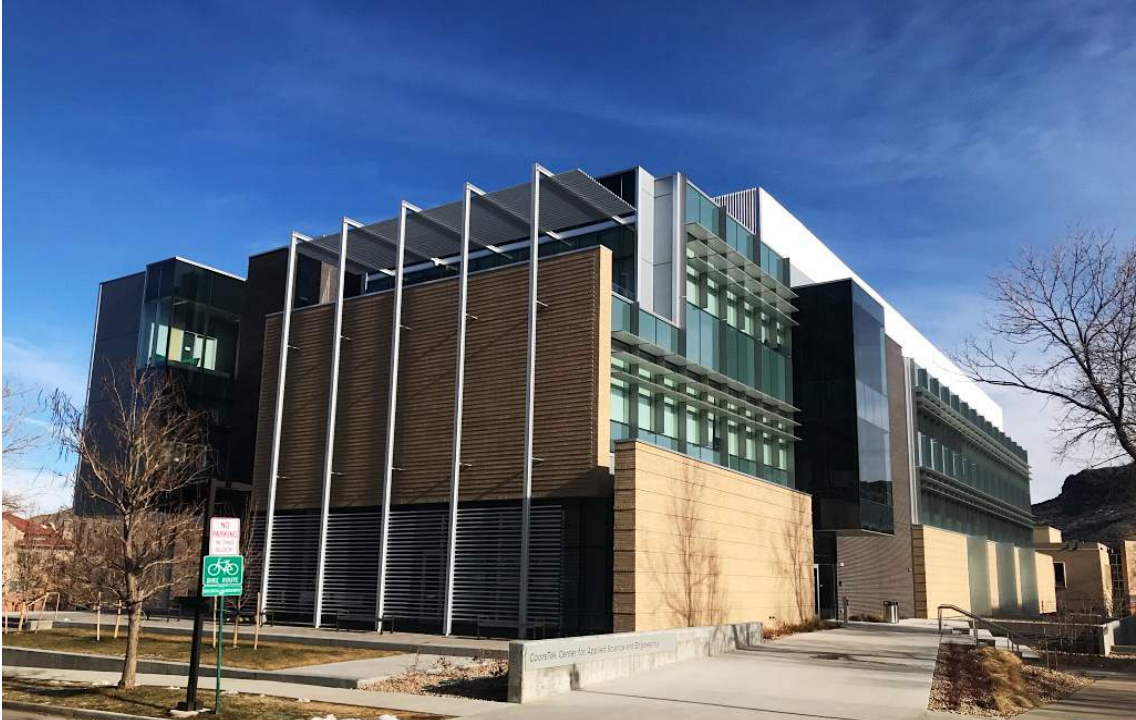
Photo 7: CoorsTek center from Illinois Street
