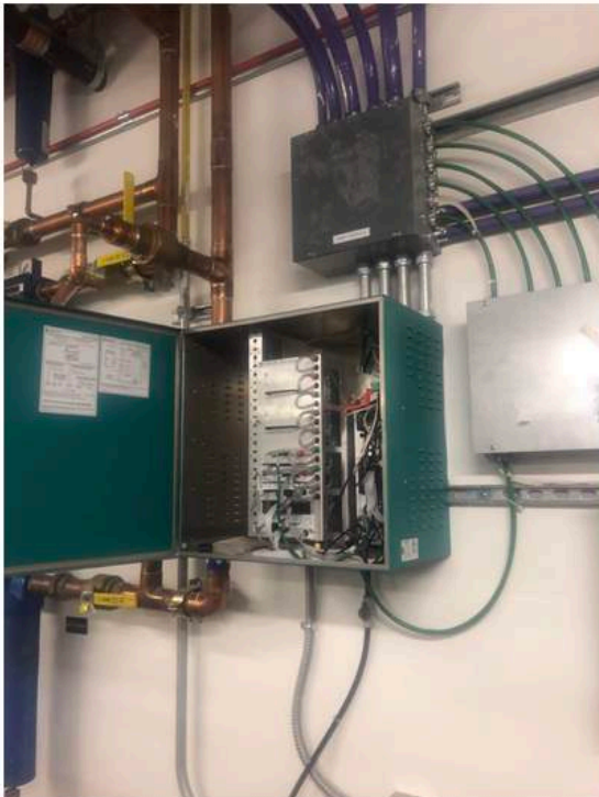
Figure 11: Lab air controller 1
