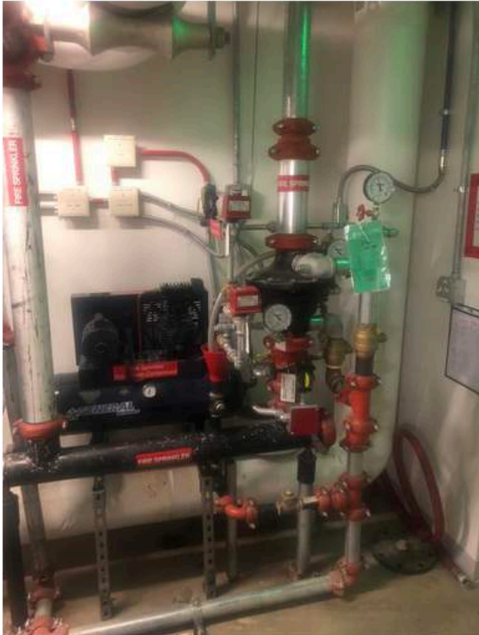
Figure 2: Fire sprinkler system
