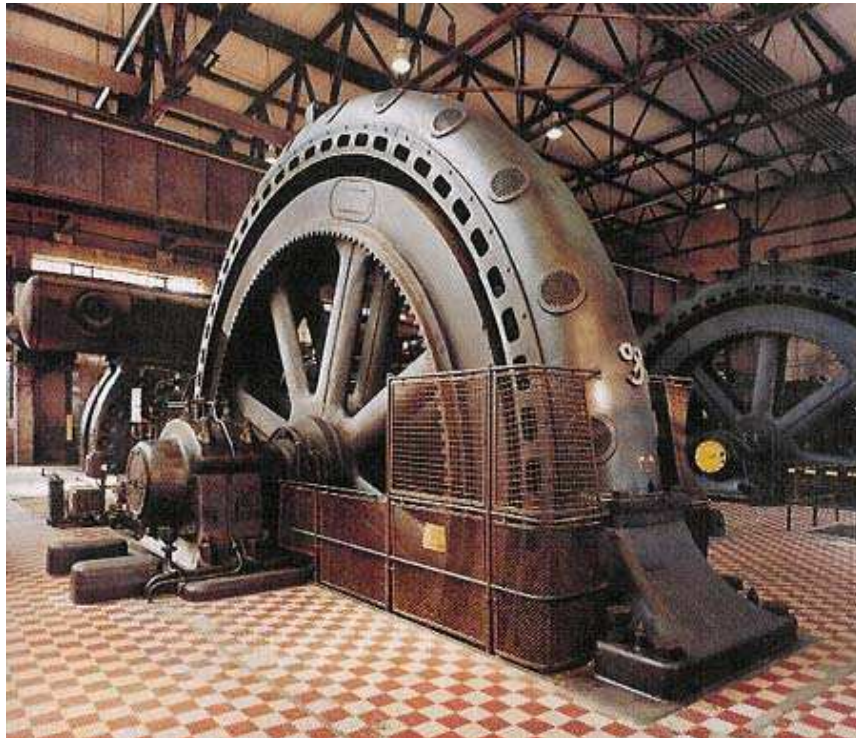
Figure 3. Example of ESS: Flywheel
