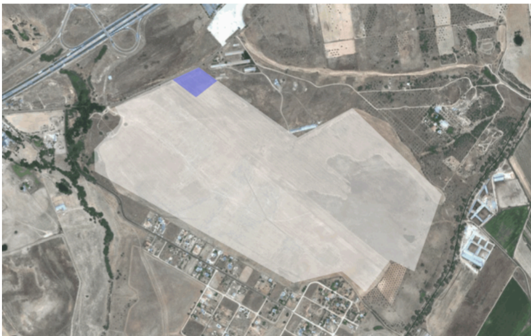
Figure 15. Area of the PV Plant in Talavera
