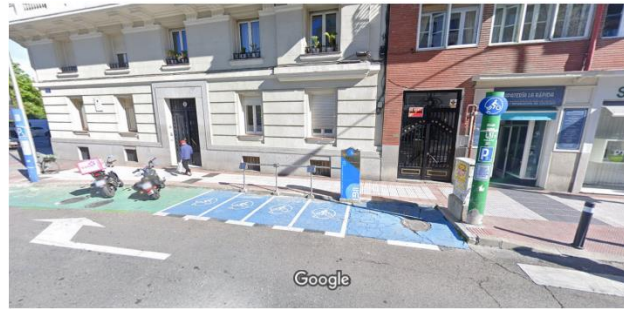
Figure 2.5 Motorcycle charging station [Google Maps]
