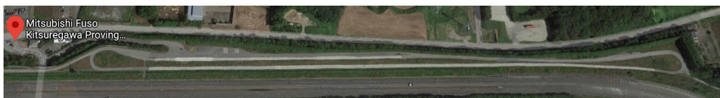
Figure 1.1: Aerial view of the Testing circuit where the model will be implemented
