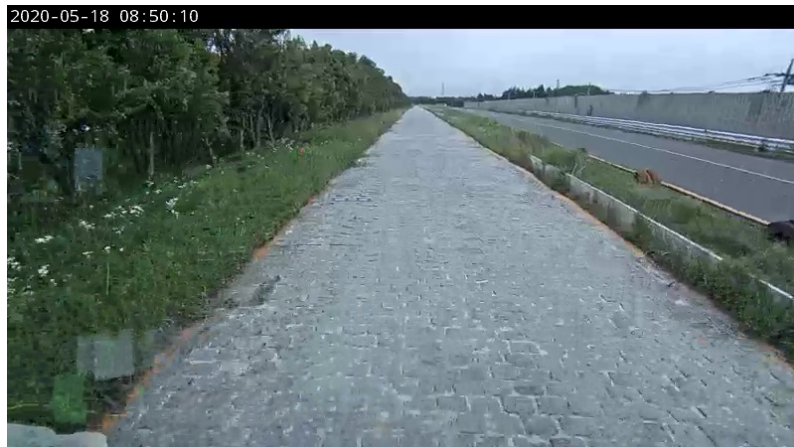
Figure 4.26: Input image before Median filtering
