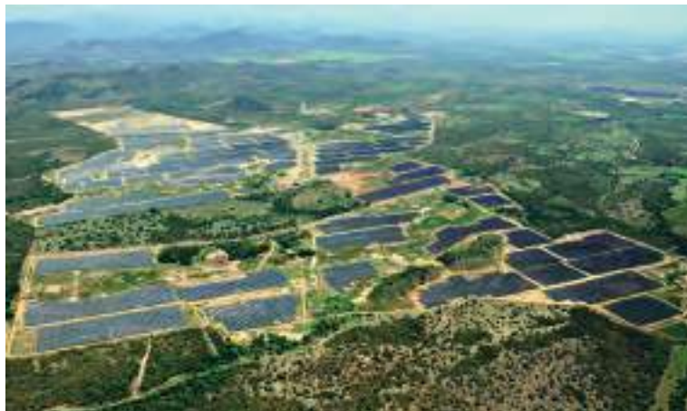
100MW solar plant located in South America.
