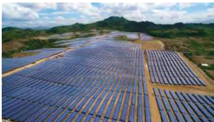
60MW solar plant located in Asia.
