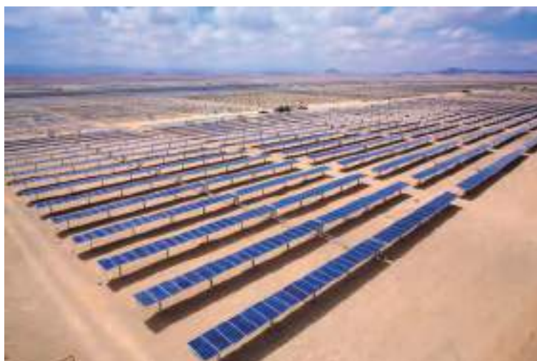
30MW solar plant located in South America.
