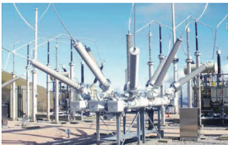
Figura 94: PASS M0S 245 kV de Hitachi
