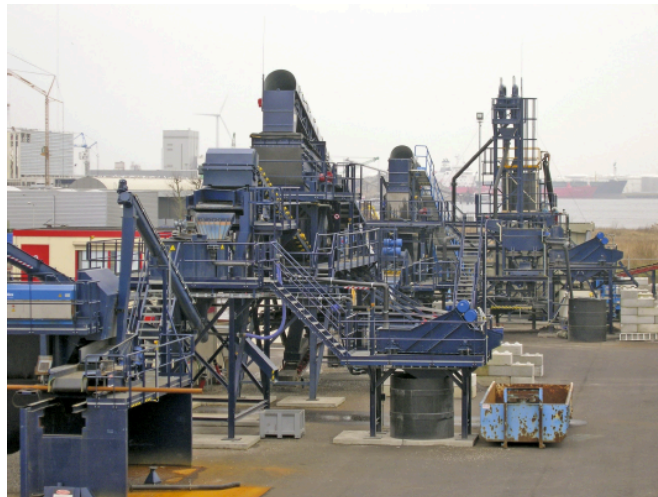
Figure 6.7: AEB Amsterdam wet separation plant
