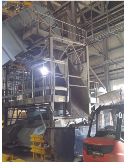
Figure 4.18: Fixed fingers screen on site and oversized container
