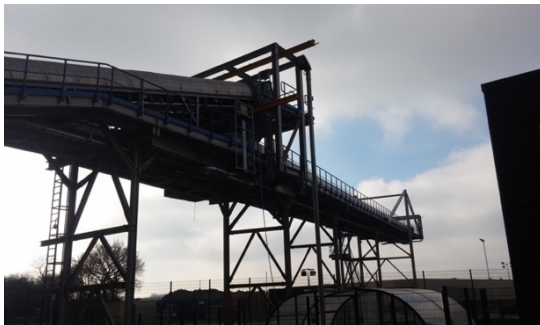
Figure 1.10: IBA Conveyor II
