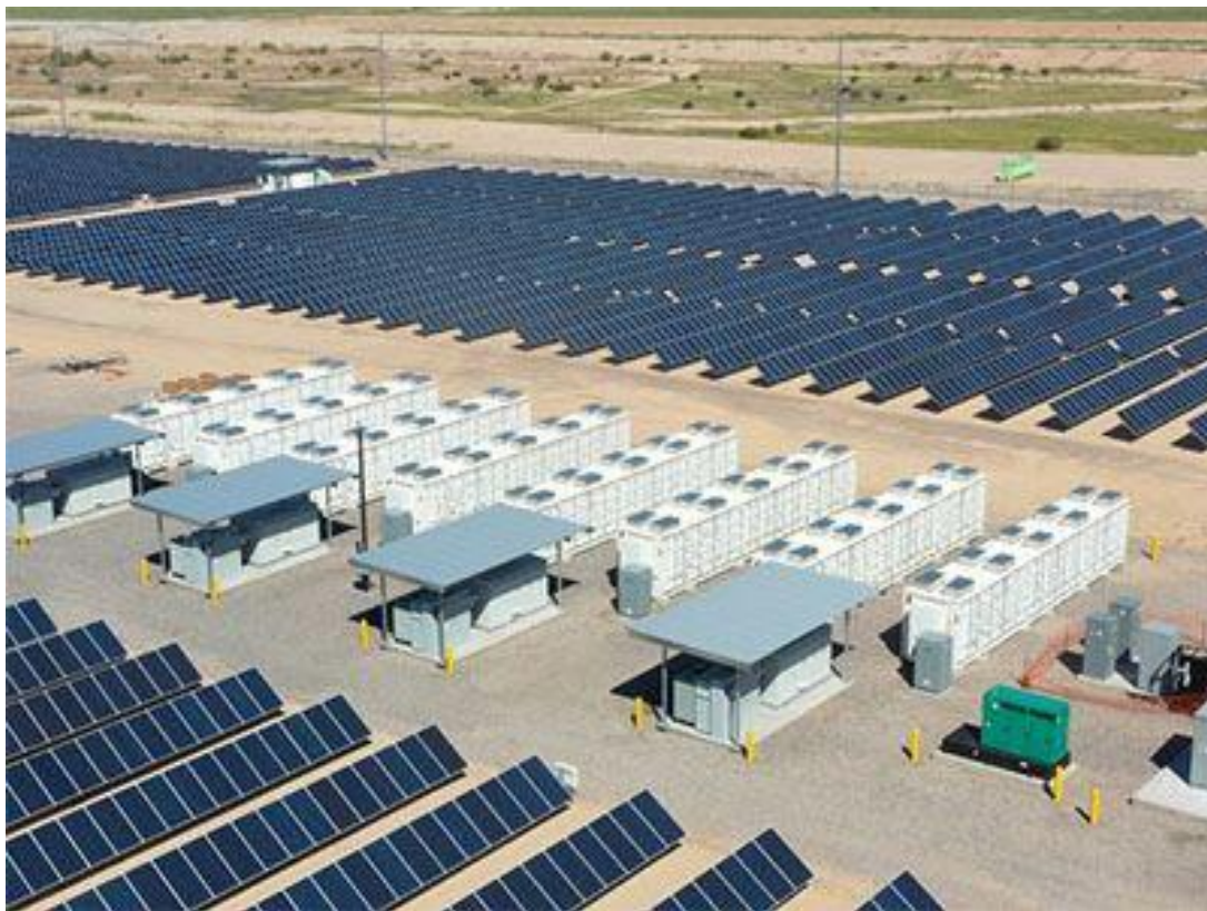
Image 1. PV + BESS coupled system
