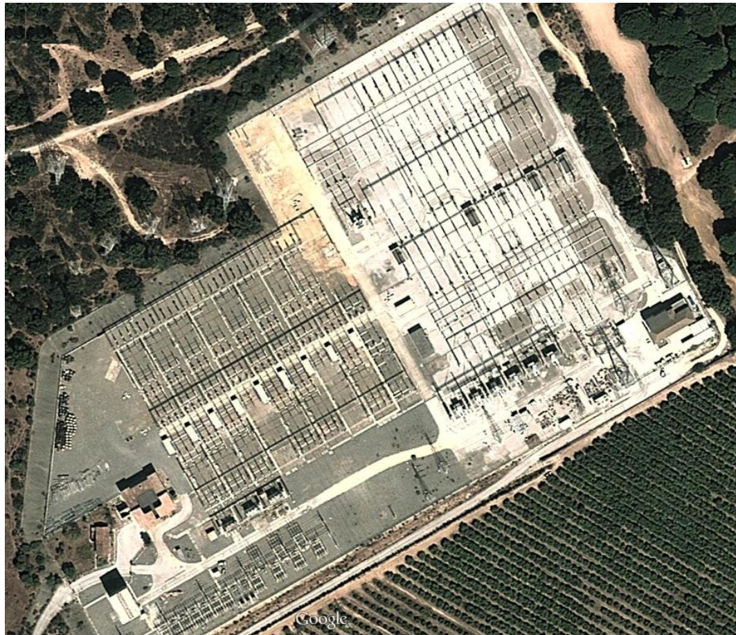
Figure 15: Aerial view of the substation Pinar del Rey (Cádiz).
