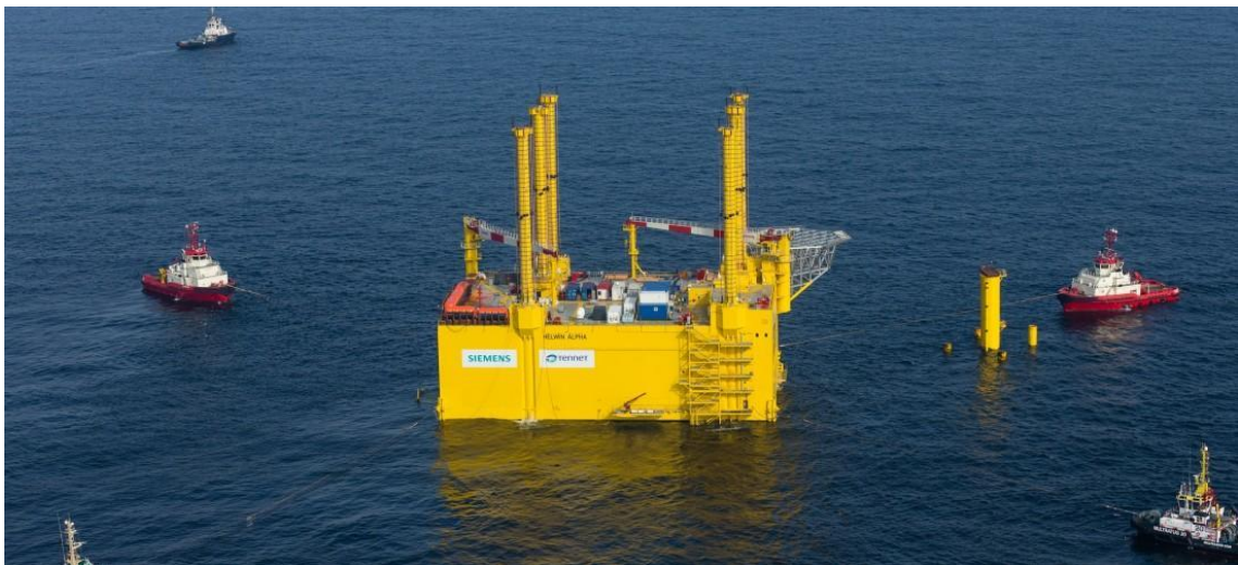
Figure 9. HVDC Offshore Platform Hel Win1
