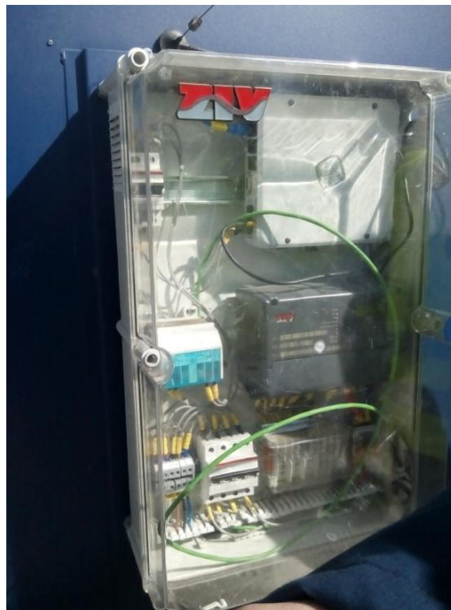
Figure 32. Remote Management System ZIV. Source: Own elaboration
