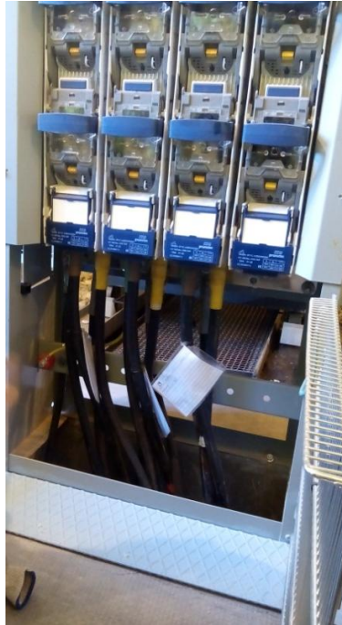
Figure 36. Low Voltage output lines/feeders. Source: Own elaboration.
