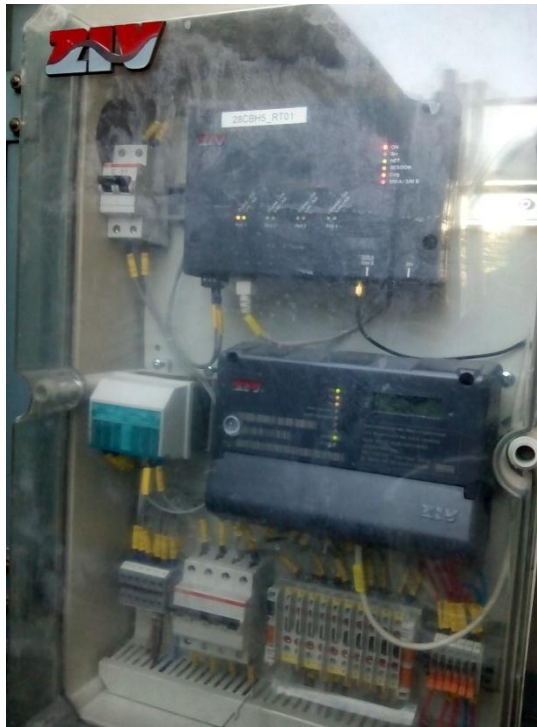
Figure 43. Remote control devices ZIV. Source: Own elaboration.
