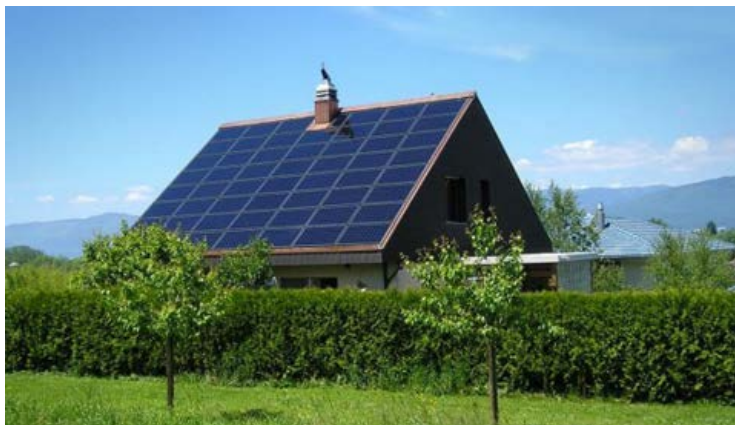
Figure 23. House PV panels rooftop integrated
