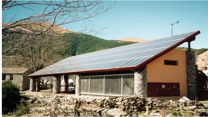
Figure 1. Centralised Photovoltaic System
