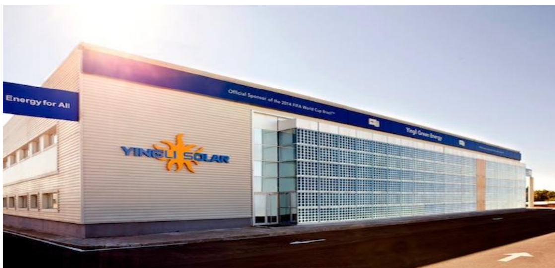
Figure 1.1 - 1 Yingli's facility in San Agostin de Guadalix
