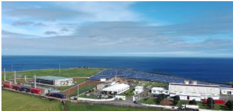
Figure 38 Graciosa PV panels, battery building and diesel power plant (courtesy of [178])
