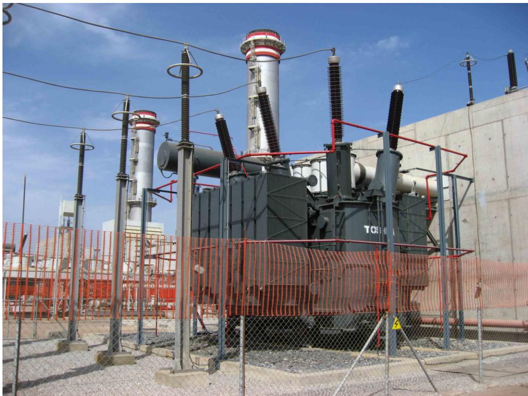
Figura 2-18-Transformador principal
