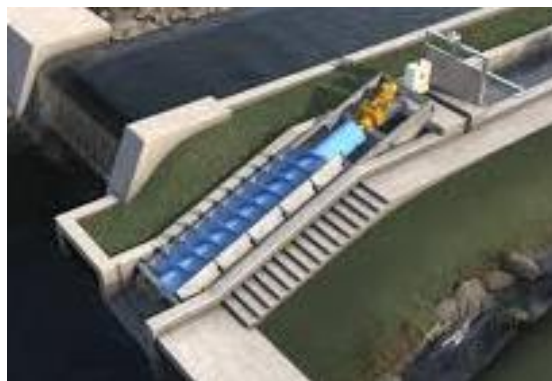
Figure 23. Screw Turbine
