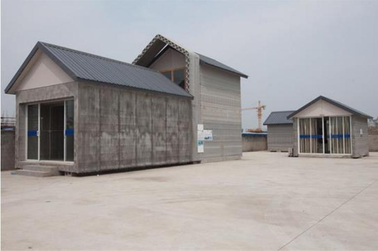
Imagen de Vivienda 3D de la empresa WinSun, obtenida de: <https://3d-expo.ru/en/article/winsun-china-builds-world-s-first-3d-printed-villa-and-tallest-3d-printed-apartment-building>
