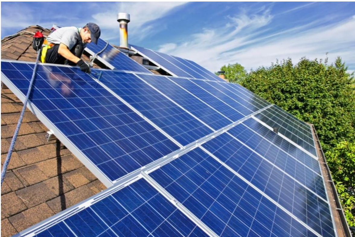
Figure 8. Solar panels installation on a house roof. Retrieved from Bloomberg.com .
