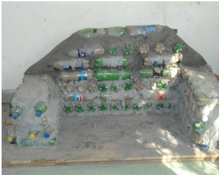
Figure 47: PET Bottle construction. Source: IRP India 2013.
