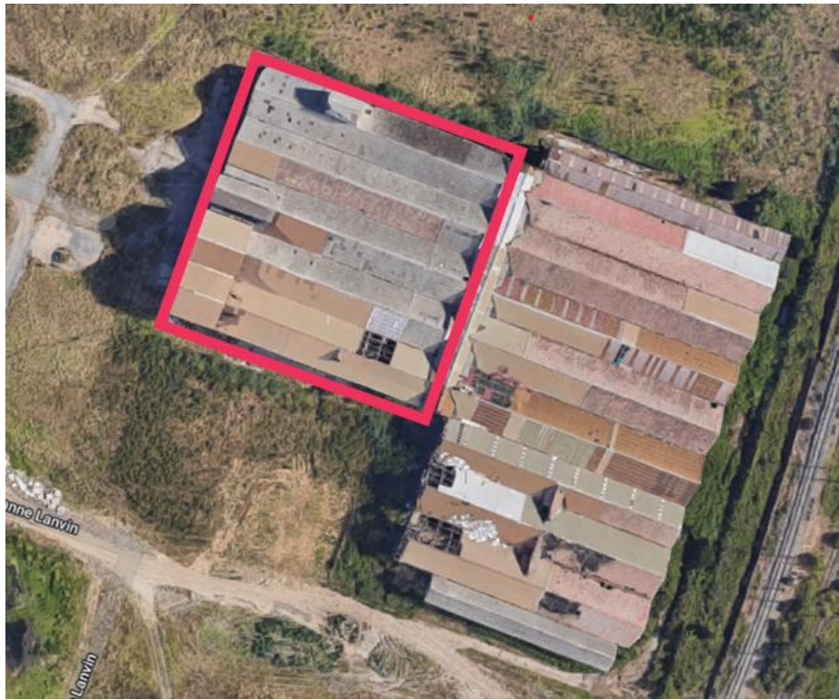
FIGURE 31 – HORIZONTAL SURFACE BEFORE CONSTRUCTION (SOURCE: GOOGLE MAPS)
