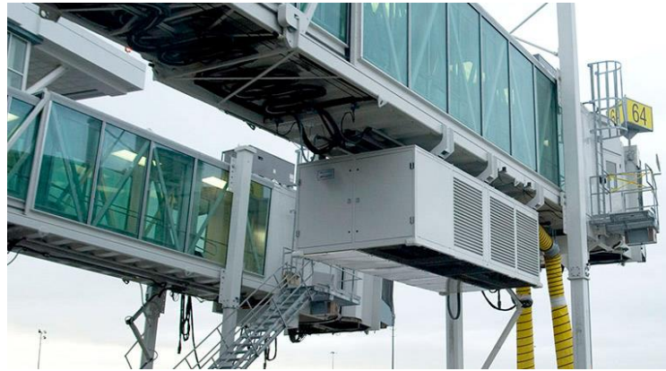
Fig 1.2. JetAire HVAC unit attached to a Jet bridge.
