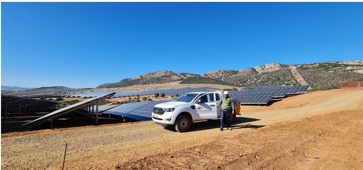
Figure 17: Solar photovoltaic panels
