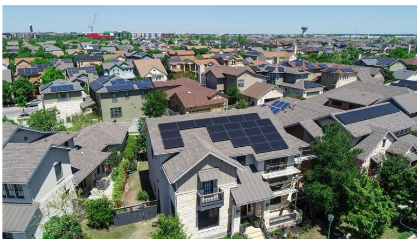
Figure 1: Solar self-consumption installation in a rooftop of a household
