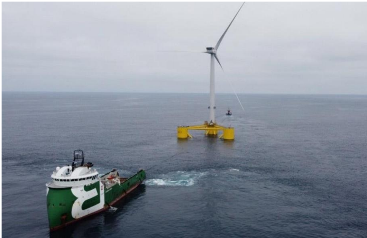
Figure 44. WindFloat Atlantic turbine installation process [48].
