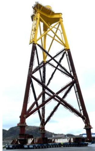
Figure 9. Jacket structure designed by Sarens [24]
