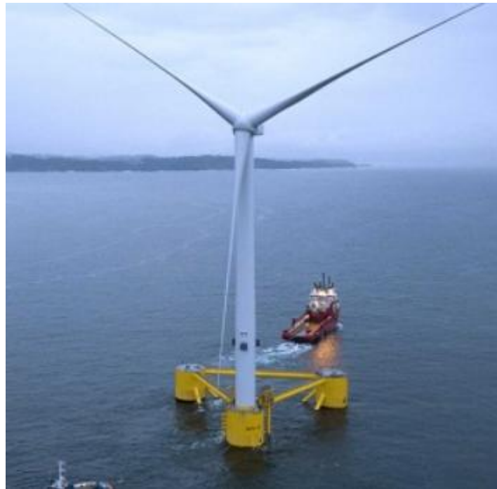
Figure 12. WindFloat Atlantic turbine in Portugal [27]
