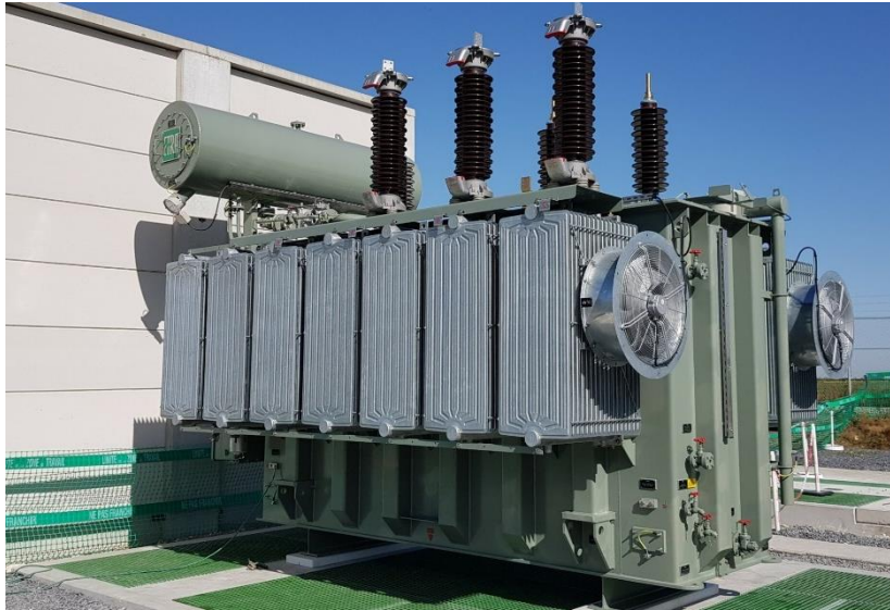
Figure 34. ONAF power transformer
