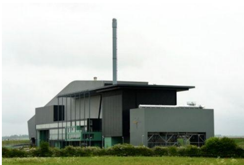
Figura 1. Planta Energy from Waste FCC, Lincoln ( resource.co )
