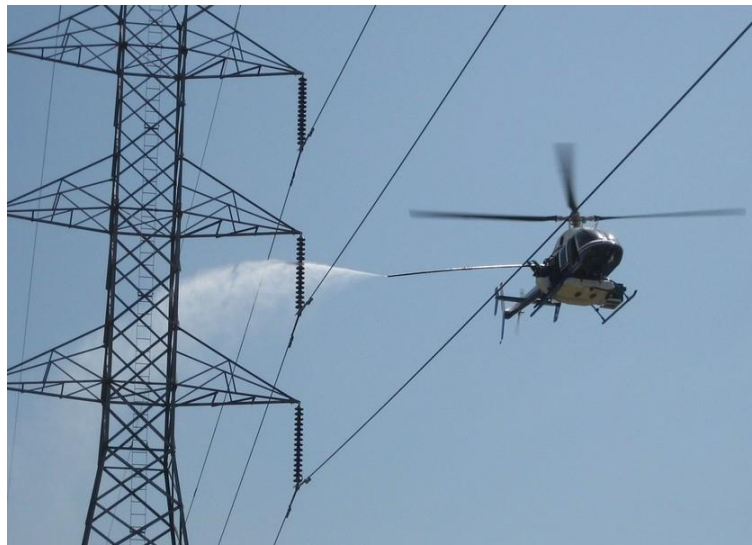
Fig. 25: Power line insulator cleaning operation [34].
