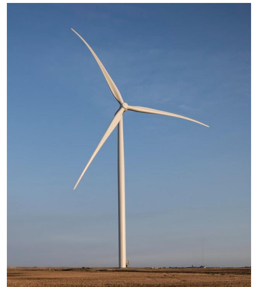
Figure 2- Three bladed HAWT (Gamesa)
