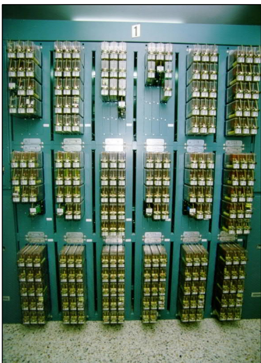
Figure 4-4. Left: Electrical Relay Interlocking. Right: Electronic Interlocking
